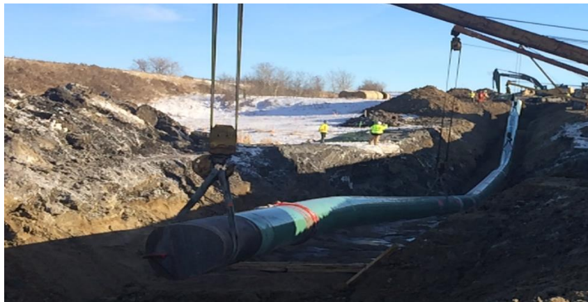
Lowering Pipe through excavated ditch at the Little Pipestone Creek
