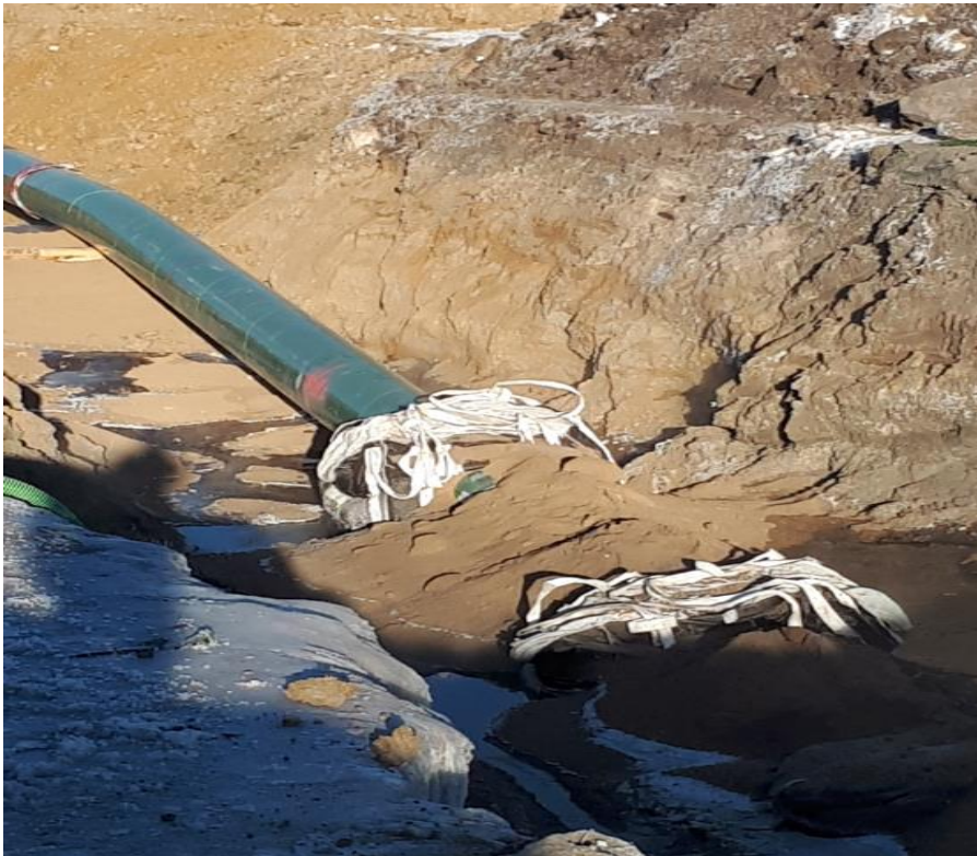
Bag weight and sand placed over product pipe
