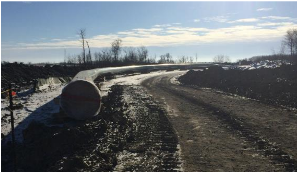
Excavated ditch through MB 1027 – 802 + 500 - pipe prepped for lowering in
