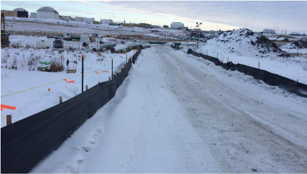
Ice bridge across the Pipestone Creek
