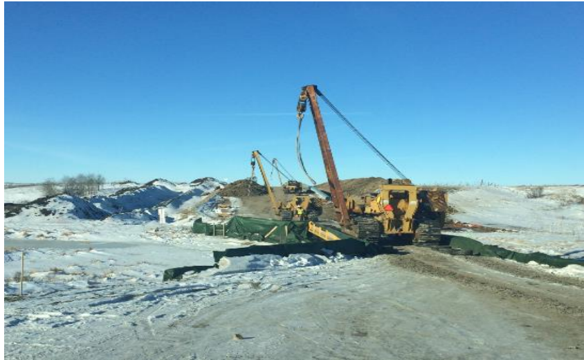
Side booms crossing Bridge at SK WC 87 Little Pipestone Creek
