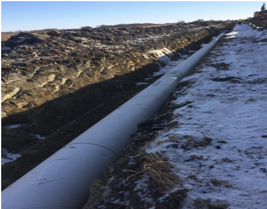
Pipe lowered into excavated ditch SK 876 Class IV
