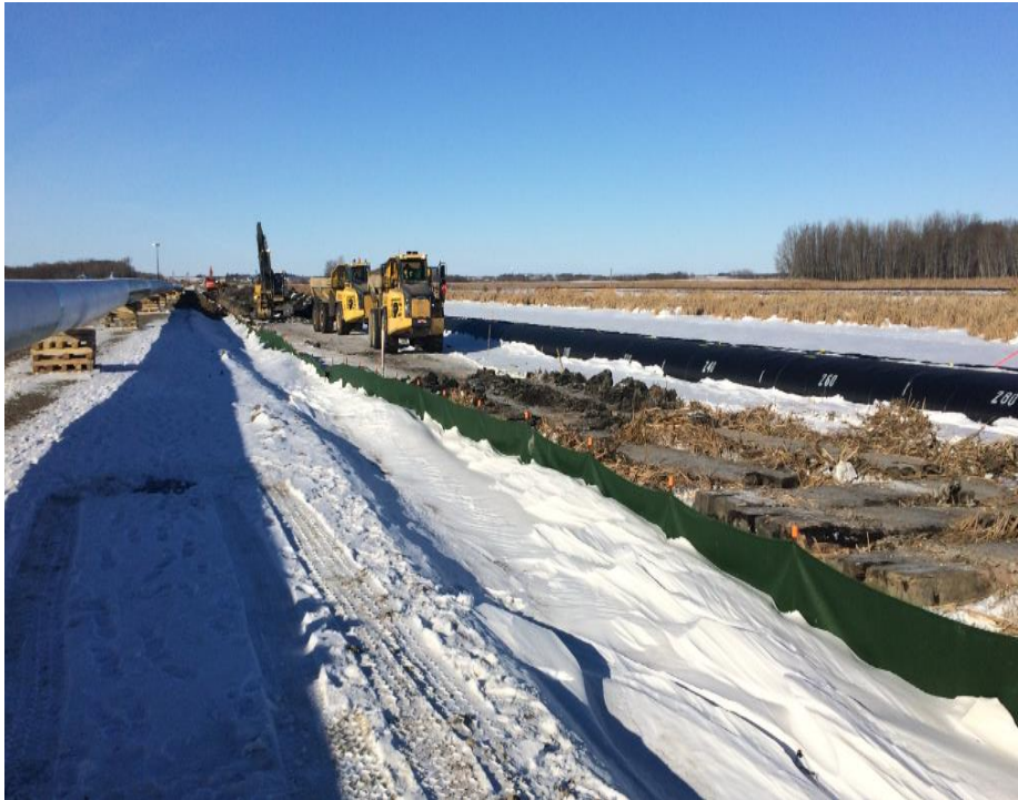
753 + 300 Excavating wetland ditch at SK 876 Class IV
