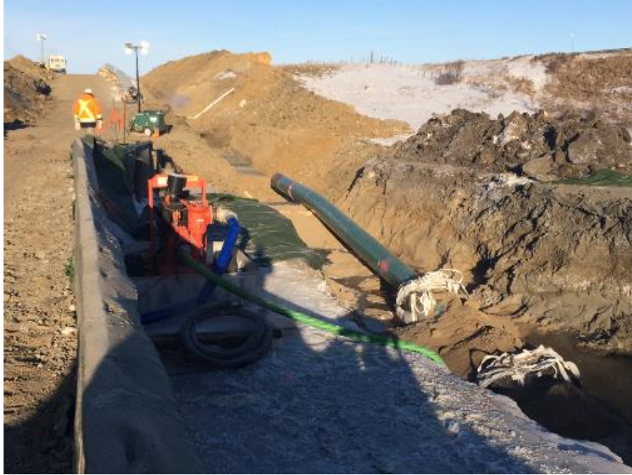
Bag weight and sand placed over product pipe
