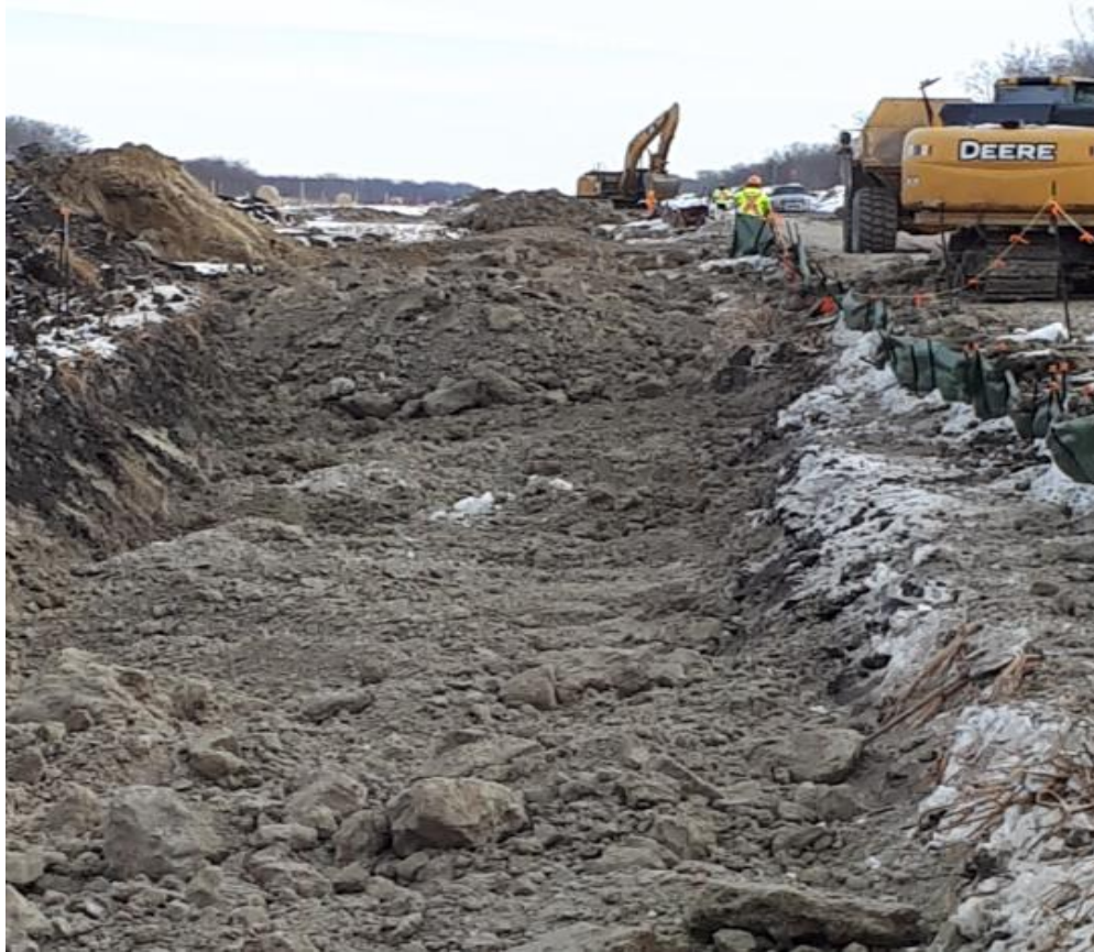
Backfilling Ditch SK 876 Class IV
