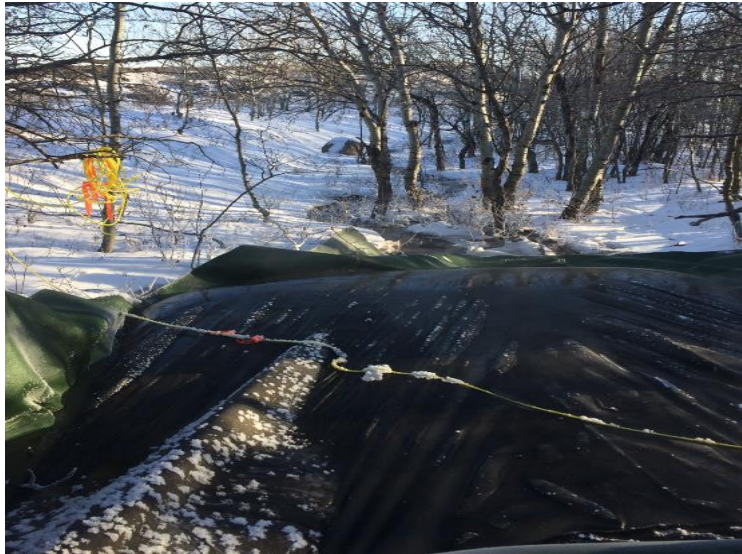
Geo teck and silk cloth placed for ground water pumped
