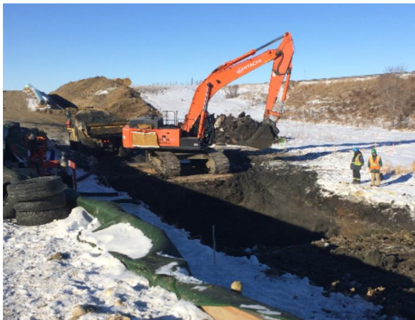
Excavating ditch line at Little Pipestone Creek SK WC 87
