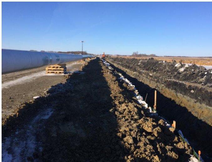
805 + 150 Ditch excavated West side of the Pipestone Creek
