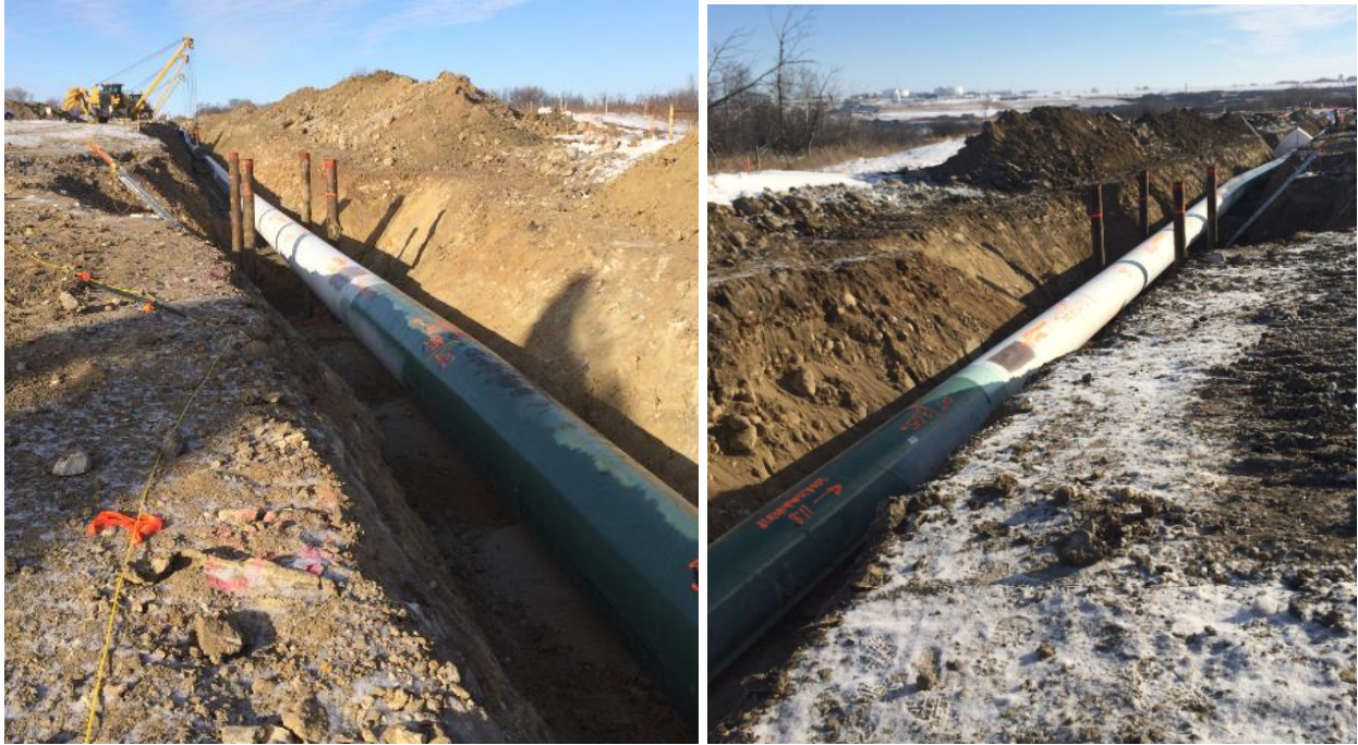
805 + 150 Sand bedding placed in ditch bottom & pipe lowered in
